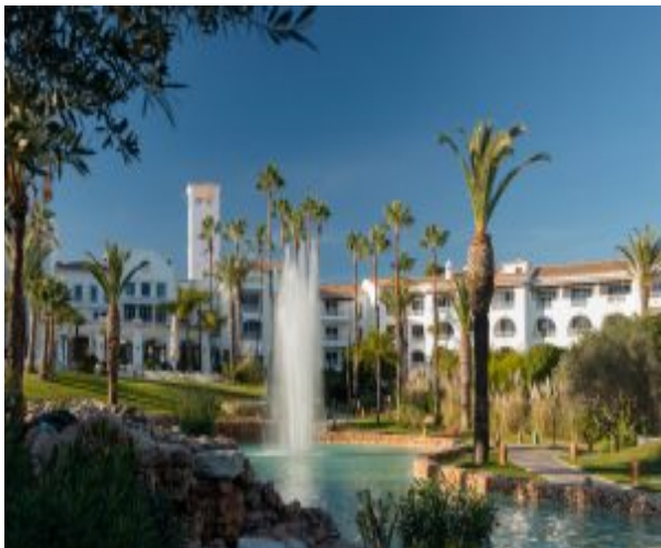
Main building and gardens
